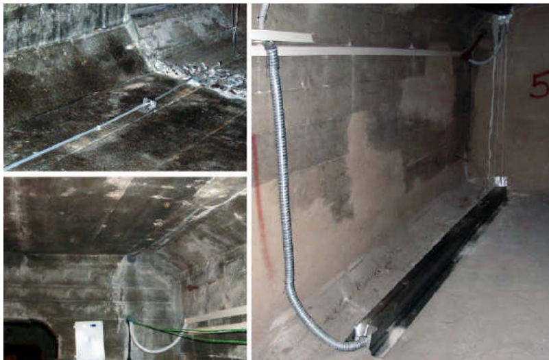
Fig. 4. SOFO sensor before (left) and after (right) protective cover was installed.
