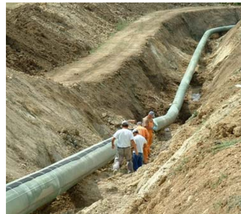
Fig. 6. SMARTape installed on the gas pipeline.
