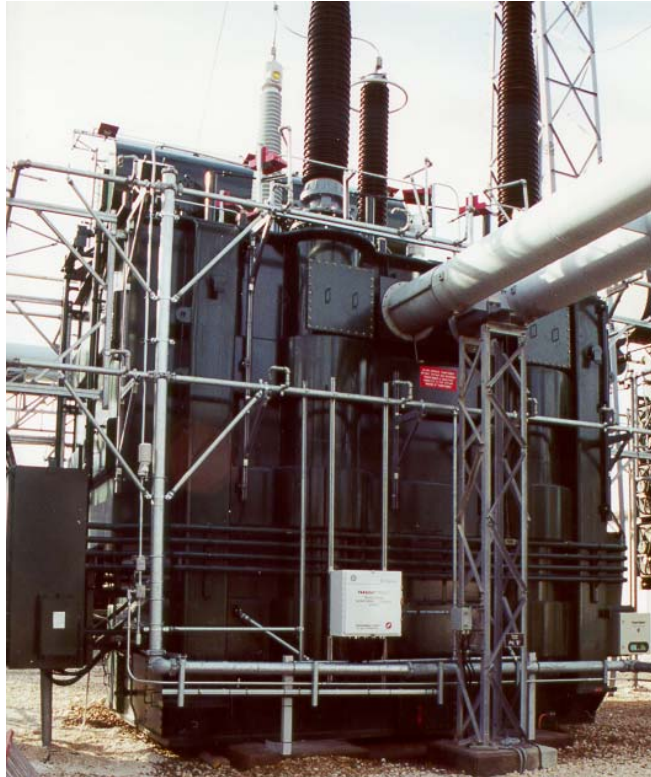
FIGURE1: Converter Transformer, 107 MVA, Single Phase
